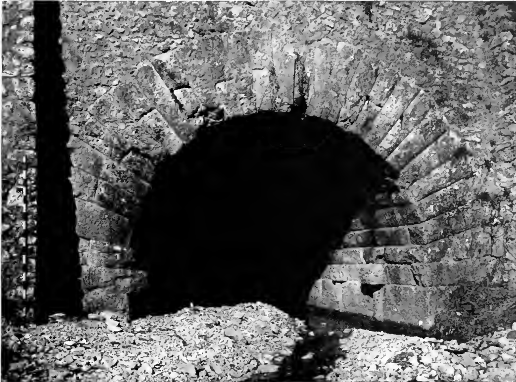
FIGURE 1. — PONTE DI SAN GIORGIO, VIEWED FROM THE EAST Only the arch of travertine is Roman
